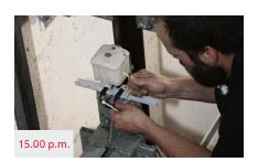
The hydraulic lift is modernized with the MULTIkit iValve
